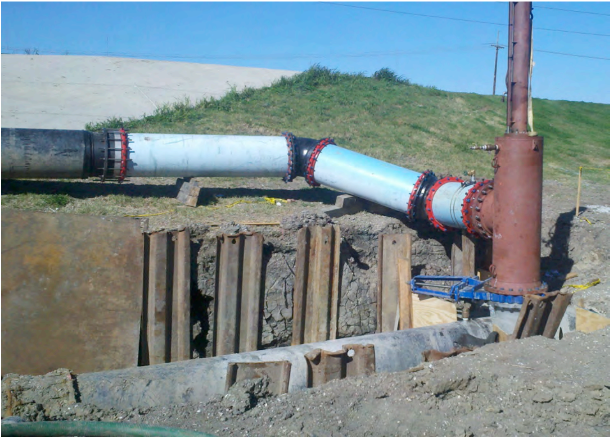
A BYPASS IS INSTALLED BETWEEN THE LINESTOPPING MACHINES.
