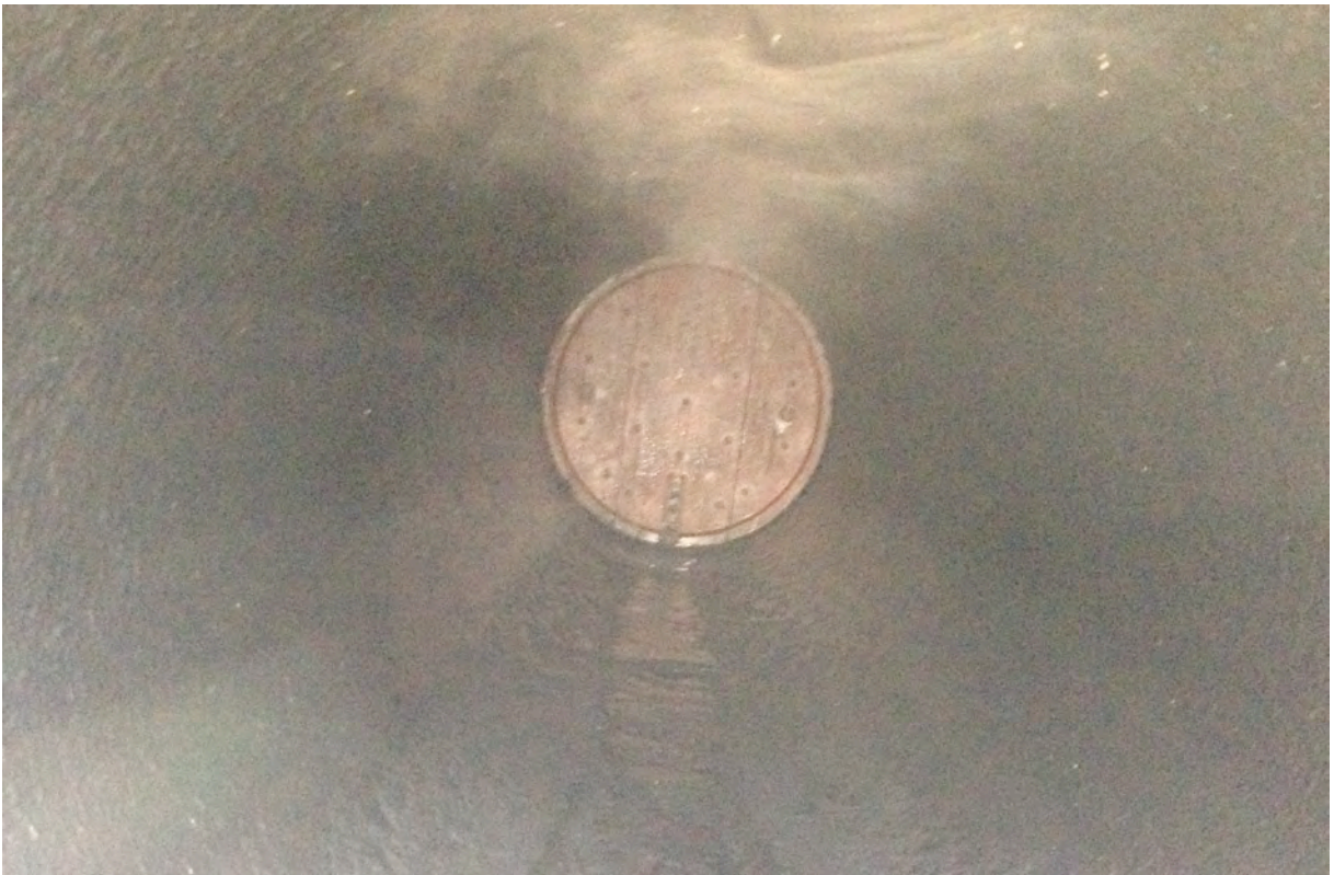
HDPE PIPE IS GENERALLY SMOOTH INSIDE SO MANY TIMES BUBBLE TIGHT LINESTOP SHUDOWNS ARE COMMON MAKING IT EASY FOR THE CONTRACTOR TO PERFORM THEIR WORK.
